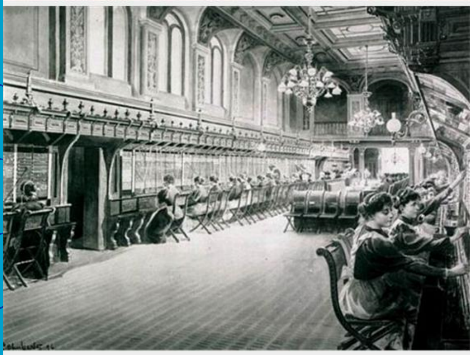
SAT's main telephone exchange, Stockholm 1897 – 7000 lines Human interaction required for cross-switchboard connections
